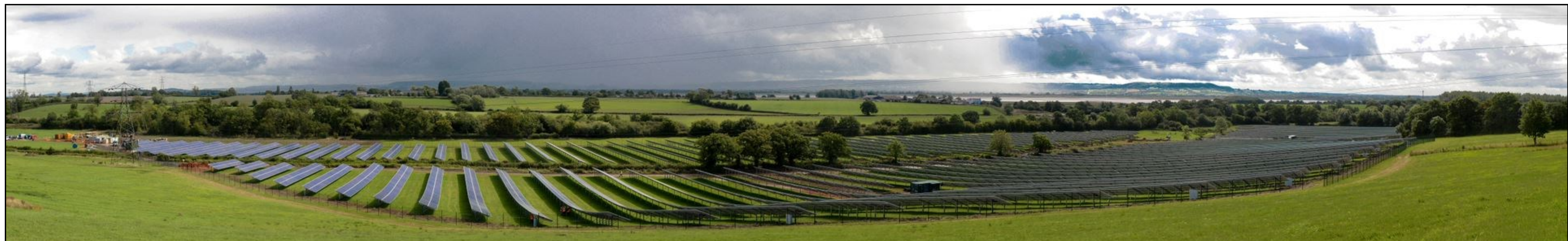
Example of Solar Array
