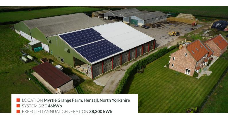
Locogen recently installed a solar PV system at Myrtle Grange Farm, a mixed livestock and arable farm near Hensall in North Yorkshire. With grain drying and cold storage resulting in high energy usage, Chris Platt, the farm's owner, was keen to find a way to reduce both his bills and the farm's environmental impact.
